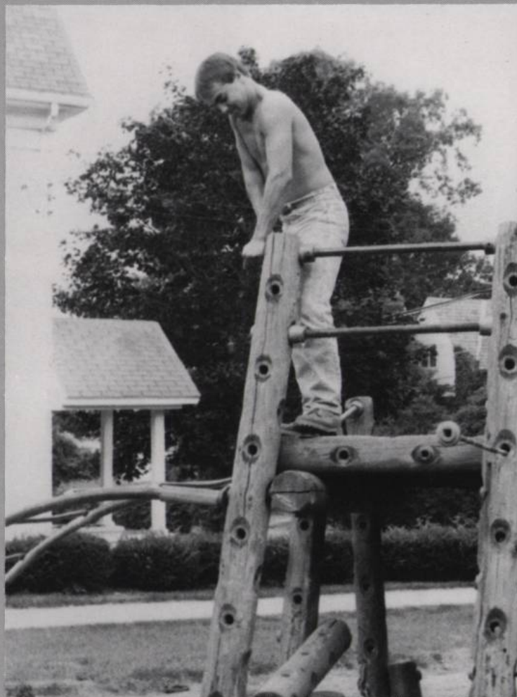
W hoops! Don't fall. Dismantling an old jungle gym is Tommy Aitken, in a Crafton park.
